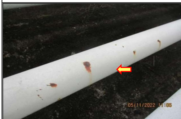
Fig.5 Minor paint damage was found however it is in acceptable condition
